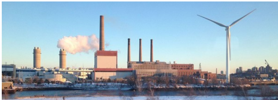
Mystic Generating Station
