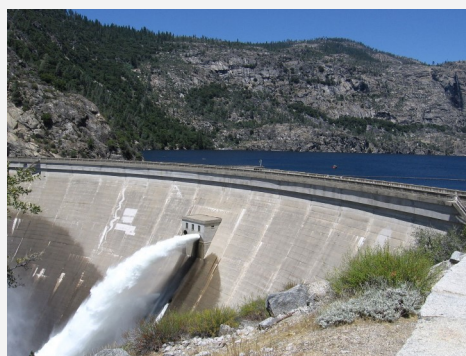
O'Shaughnessy Dam, part of the Hetch Hetchy Project
